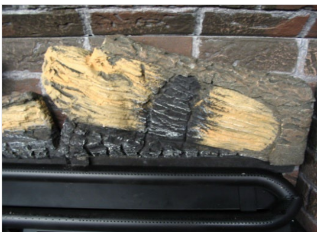
Log "B" installed correctly
